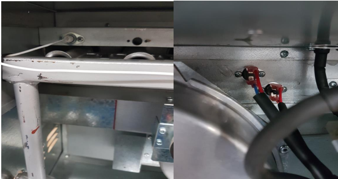
Photograph 3- Location of the flame sensor
