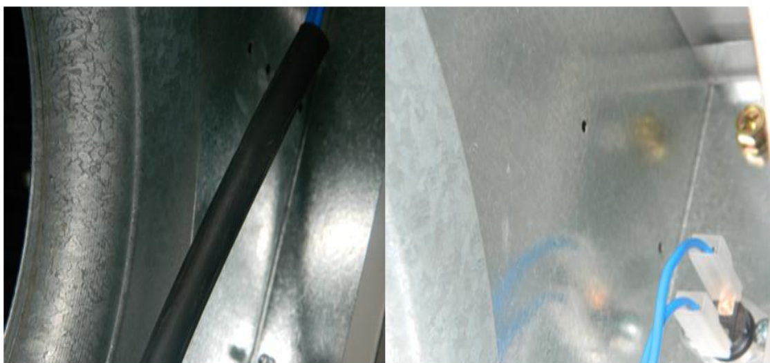
Photograph 1- Location of the fan side auto resettable A60 over temperature switch, one each side
